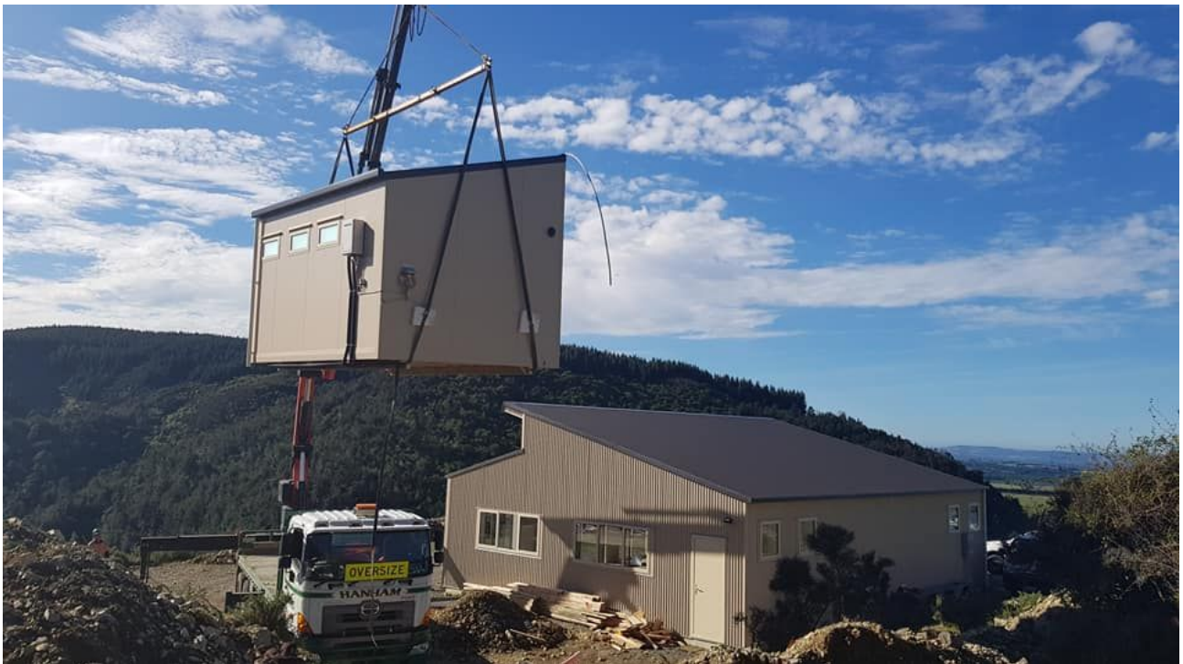
Installation of a toilet and shower block, 2018
