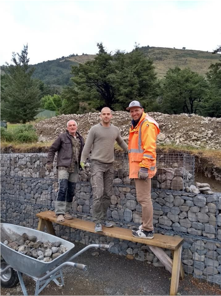
Building gabion retaining walls around gompa and toilet block
