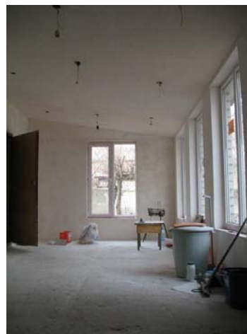
We made the ceiling and finishing works in the verandah...
