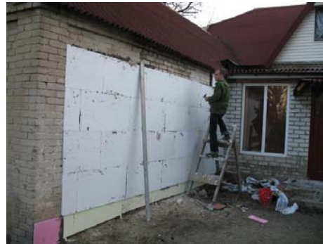
Partially made warmth keepers in the house walls.
