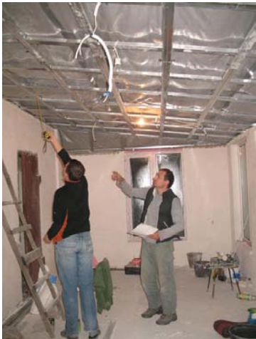
We made twofold warmth keeping the ceiling in the verandah.
